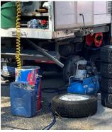
Spill trays under fuel drum and generator are not in place.
